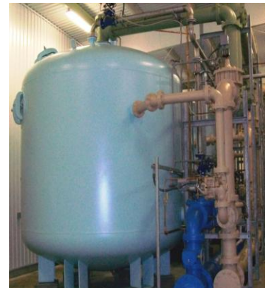
Typical Vertical Pressure Filter
