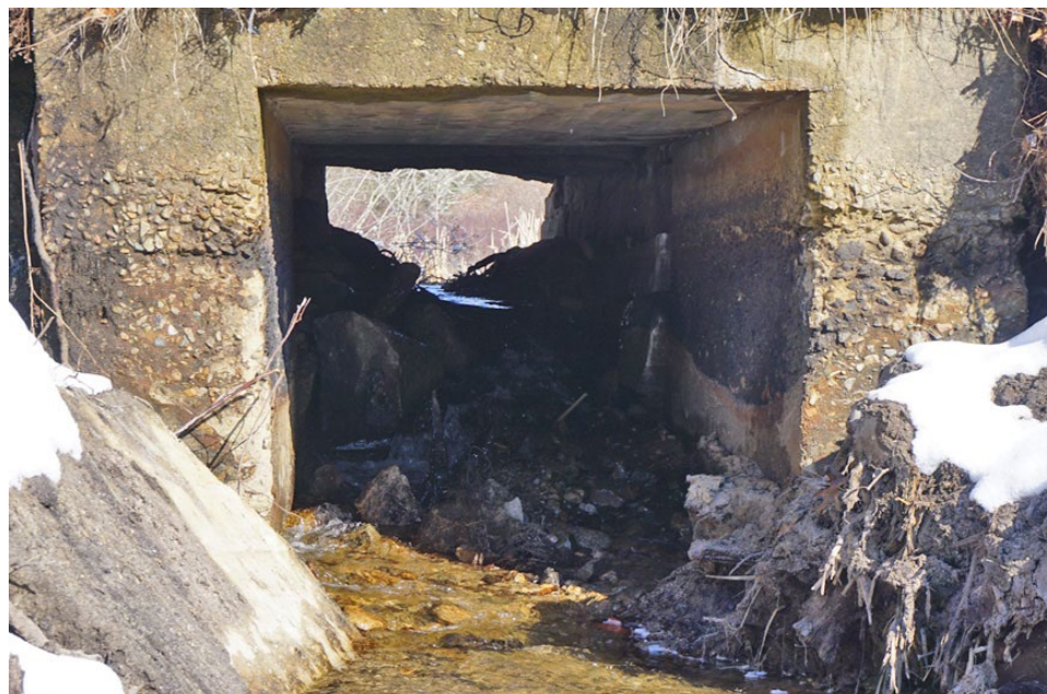
Clogged / Deteriorated Culvert
