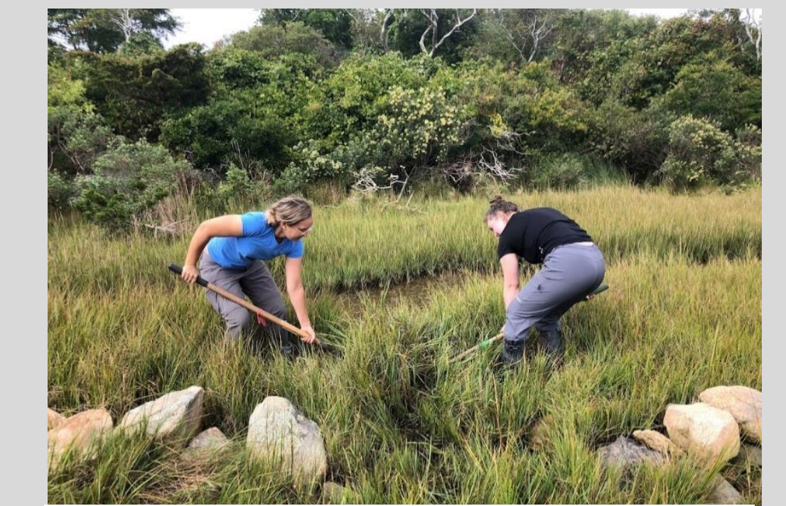
Removal of section of stone wall and installation of runnel
