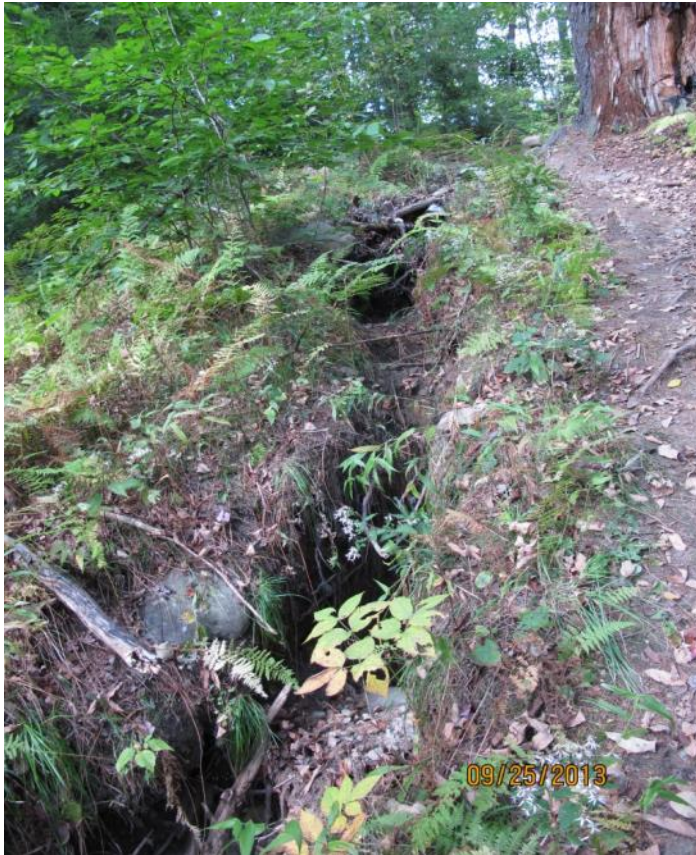
At Drainage Outfalls
