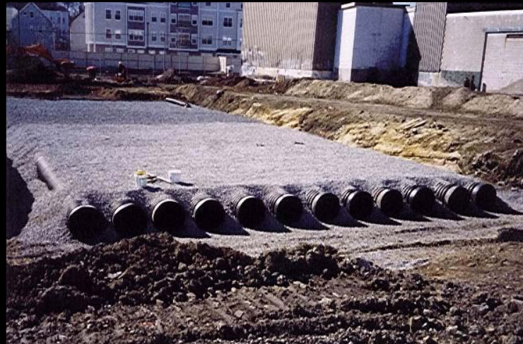
Underground Infiltration
