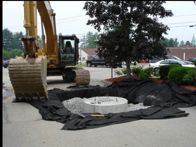
Leaching Catch Basins/Roof Leader Dry Wells
