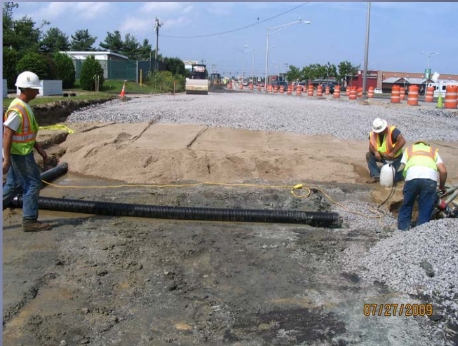
Maine Mall Road - Construction 7/27/2009
