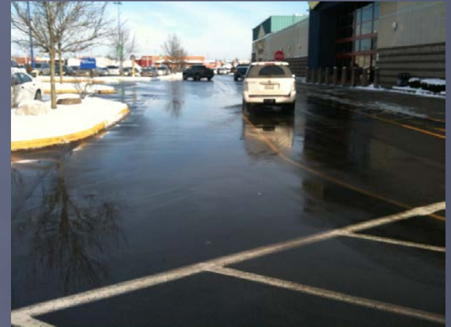
Maine Mall Parking Lot 1/17/2013
