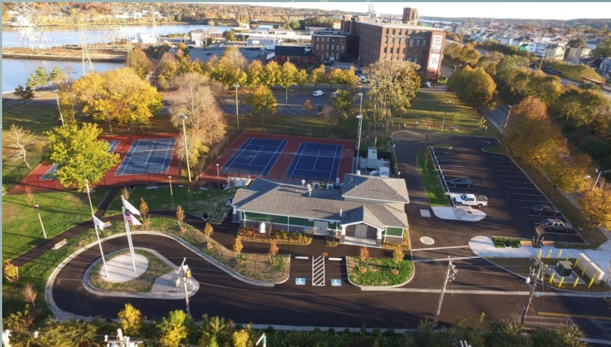
President Ave CSO Screening and Disinfection Facility
