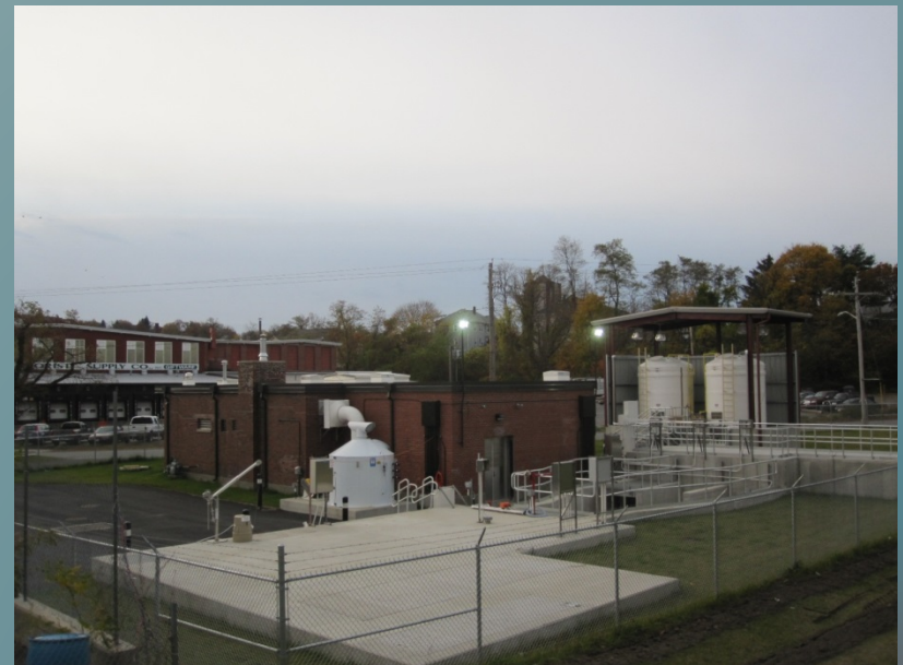
Cove St. CSO Screening and Disinfection Facility
