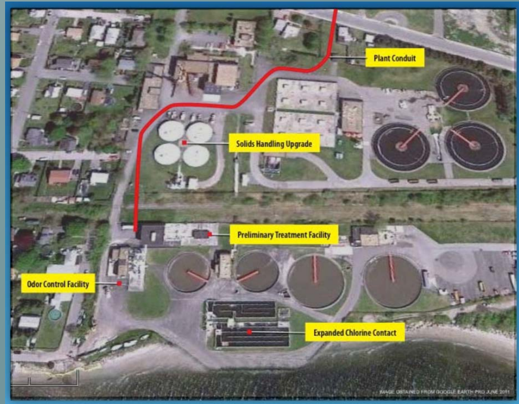
Image source: CSO Abatement Program Update, City of Fall River
