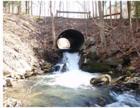
Figure 20. Perched culvert beneath Ryan Road.
