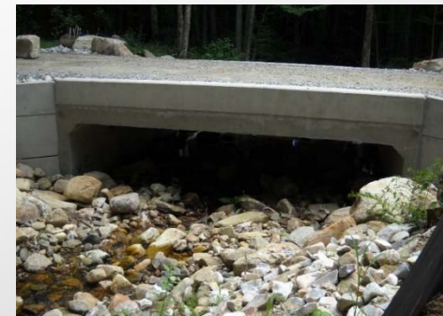
Figure 20. Perched culvert beneath Ryan Road.
