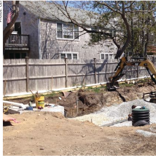
Hyannis Inner Harbor BMP during construction
