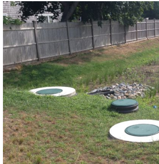
Completed Hyannis Inner Harbor BMP
