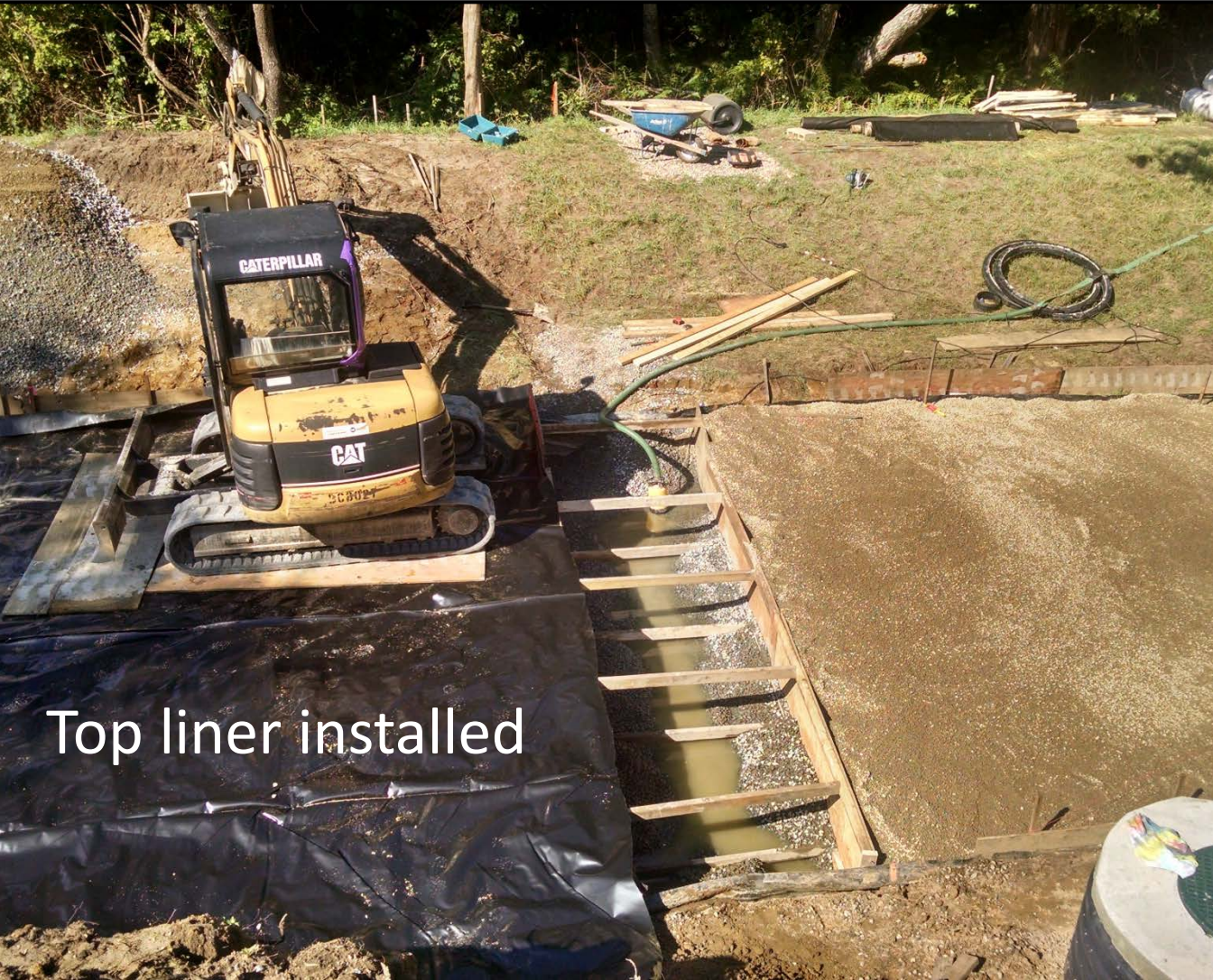
Bio-soil installation
